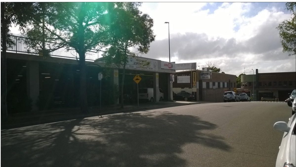
Plate 4: the south-eastern section of the site viewed from across Pritchard Street, showing the undercroft and roof-top parking areas.
