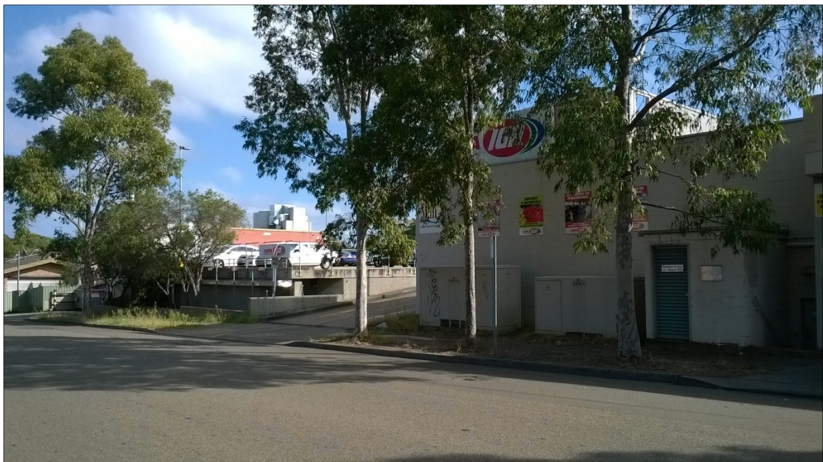
Plate 2: the shopping mall viewed from across Pritchard Street showing the electrical substations.
